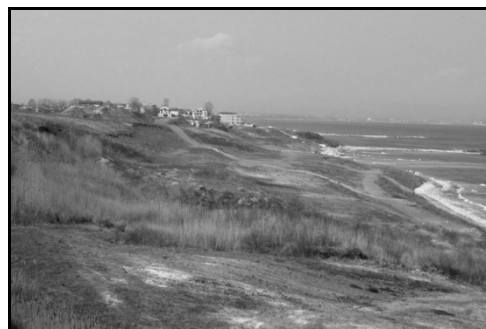
Fig.3 The sea front affected by landslides in the South of Tuzla
