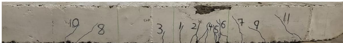
Fig. 5d. Crack Propagation of RC beam using Steel bars and PVA fibers (S30 0.25PVA)
