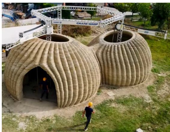
Fig. 5. WASP (Italy’s pioneering specialists in 3D printing) has completed the printing phase of the TECLA supporting structure, the first and unique fully 3D printed construction based on natural materials and made with multiple 3D printers operating at the same time. The innovative habitat model engineered by WASP and designed by MCA - Mario Cucinella Architects was conceived as a new circular model of housing entirely created with reusable and recyclable materials, sourced from local soil, carbon-neutral and adaptable to any climate and context. Source: Alfredo Milano, CC BY 2.5 < https://creativecommons.org/licenses/by/2.5 >, via Wikimedia Commons
