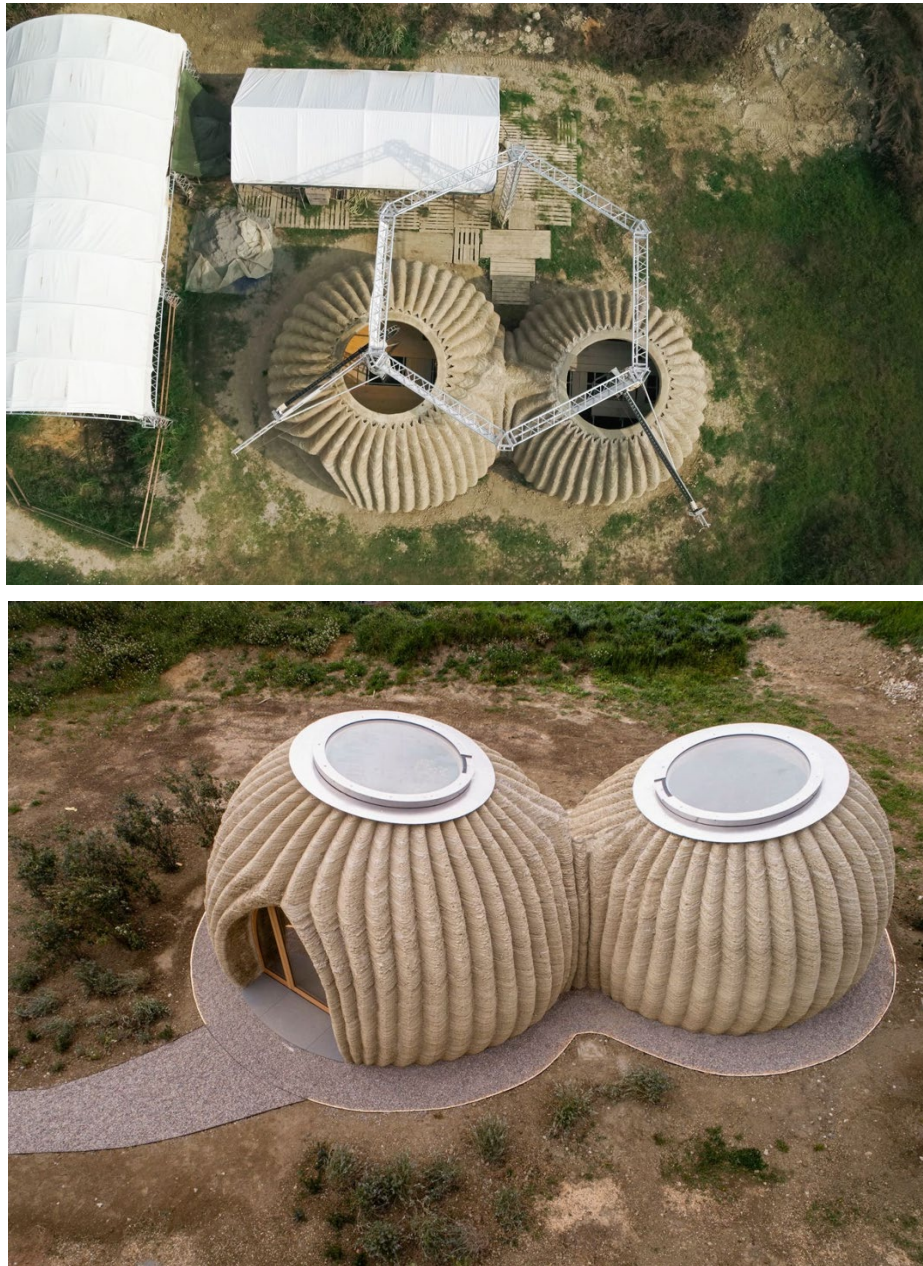
Figs. 8. 9. TECLA by Mario Cucinella in collaboration with WASP. View of On-site 3D printing in Massa Lombarda, province of Ravenna, Italy
